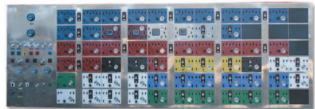
Injection Rate Control Panel
