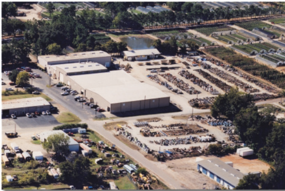
Tyler, Texas: With 100,000 square feet under roof, the seven acre facility has ten overhead cranes (including two 25 ton) and a 26 foot hook height.
