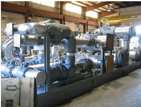
Intercooler Water Circ. Package Customer: GE/Basin Electric
