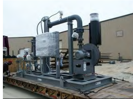
Ammonia Flow Control Package Customer: Sunoco Refinery
