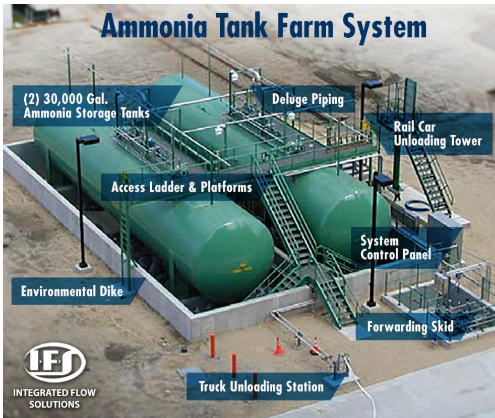
ABOVE: Exmple of an Ammonia Tank Farm built by IFS.
